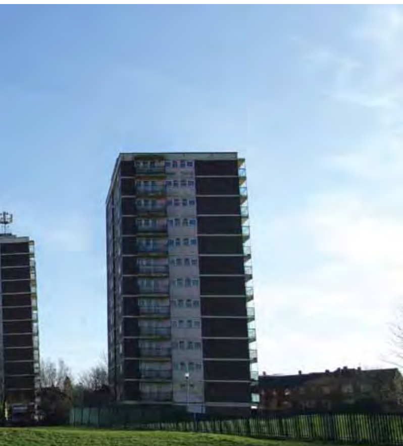
...ing the go ahead for demolition of the tower blocks.
